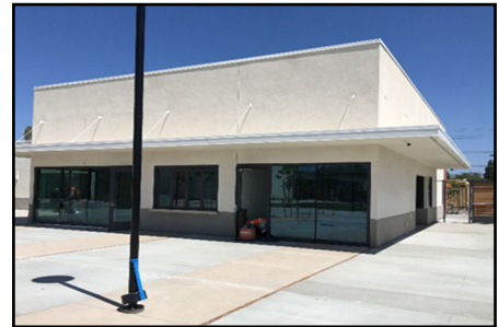
Parish Center from Courtyard.
