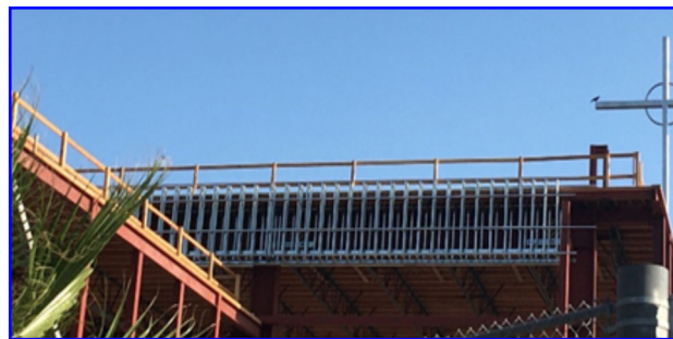
Framing for the Parapet on the Church roof
